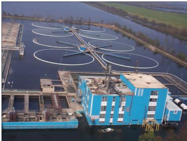
FLOODING AT EAST BANK WASTEWATER TREATMENT PLANT
