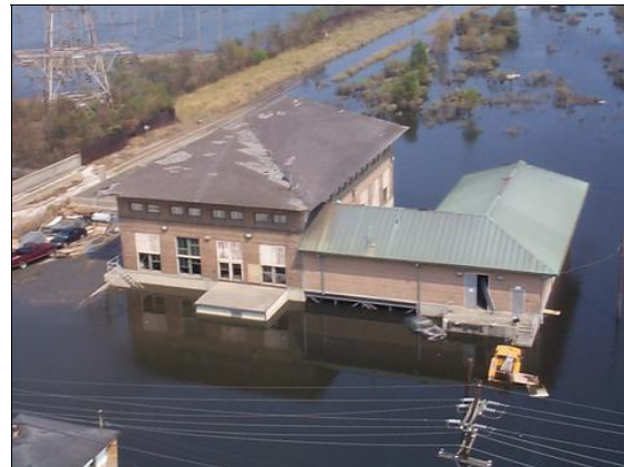
S&WB'S DRAINAGE PUMP STATION #5
