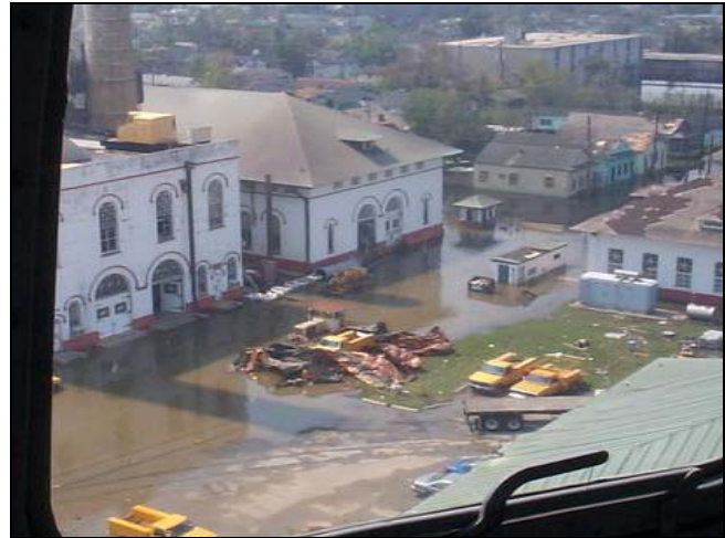
FLOODING AT CARROLLTON POWER PLANT
