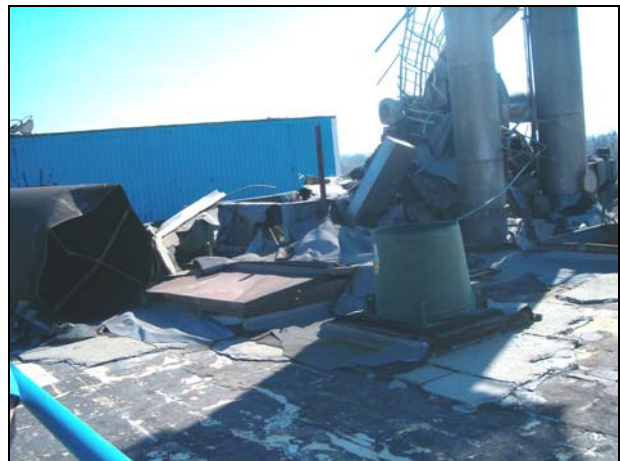
WIND DAMAGE TO ROOF AND STACK AT EAST BANK WASTEWATER TREATMENT PLANT
